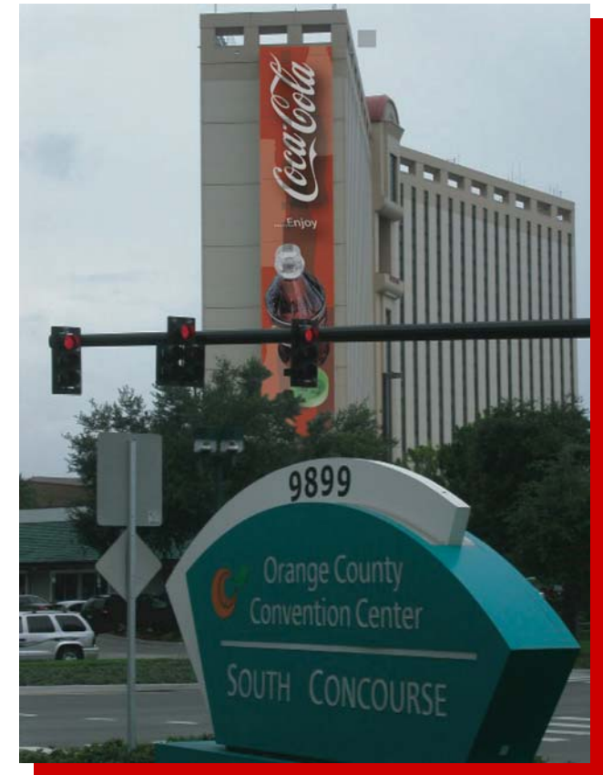
South Concourse Facing Wall
